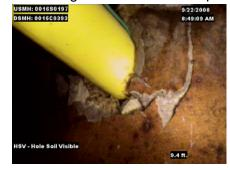
Many gas utilities are requiring an increasing level of prevention during new construction activities. The process usually requires entering the existing sewer lines with cameras attached to sondes. The sondes transmit a radio frequency that can be received at ground elevation and report the horizontal position and approximate depth.
