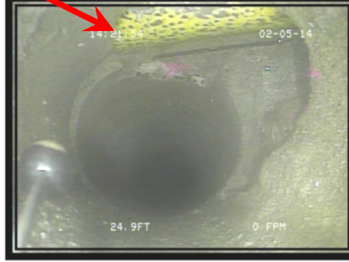
Interior Pipe Photo
