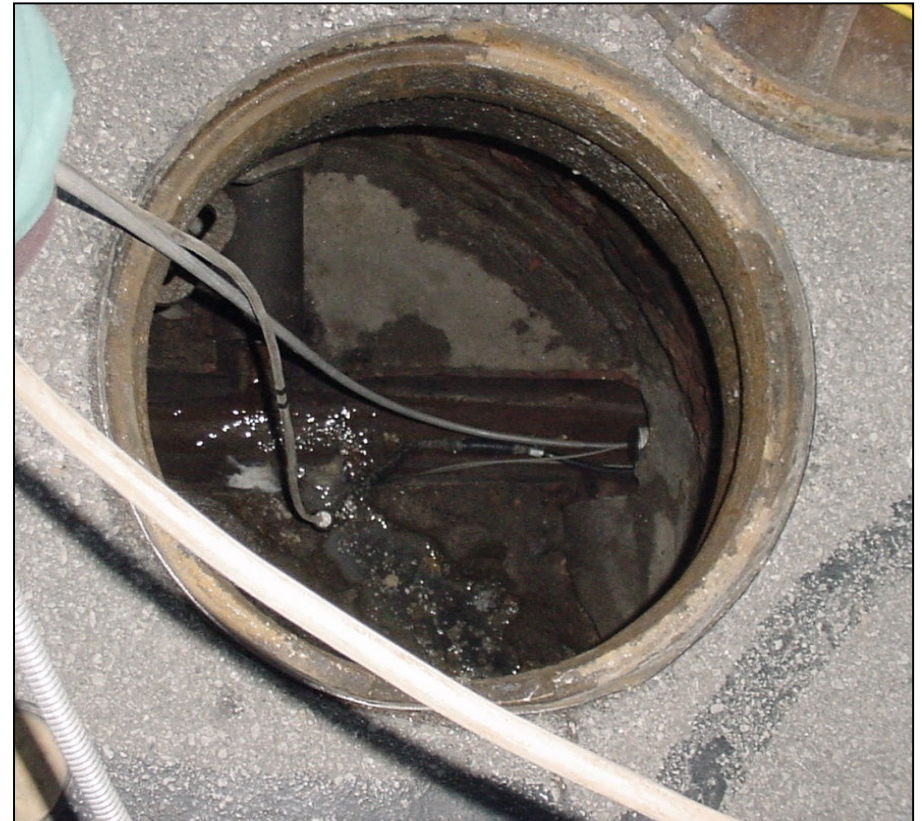
Traveling in Sewer Line
