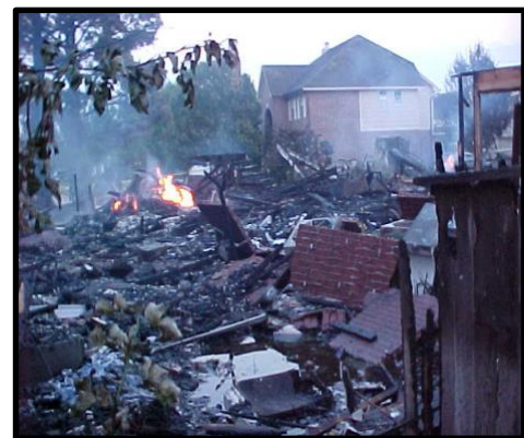
Figure 5: Results of Class 2 Cross Bore Explosion, Texas
