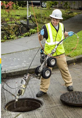
A technician with PSE service partner Hydromax USA places a robotic camera down a sewer to inspect for a natural gas pipeline, visible on the monitor below.
