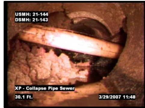
Figure 3b: Cross bores of Sewer.
