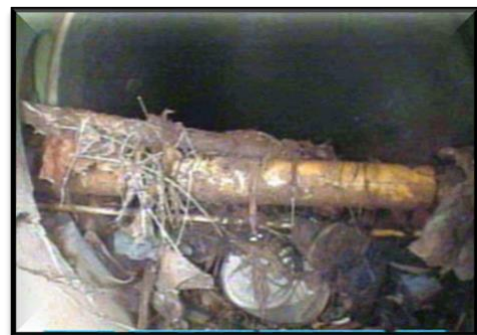
Figure 3a: Cross bores of Sewer.
