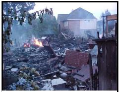
Figure 5: Results of Class 2 Cross Bore Explosion, Texas as shown in Fig. 4
