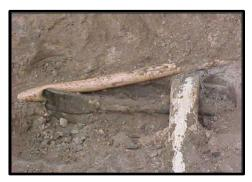
Figure 4: Class 2 Cross Bore. New communications HDD intersects sewer lateral then gas distribution line
