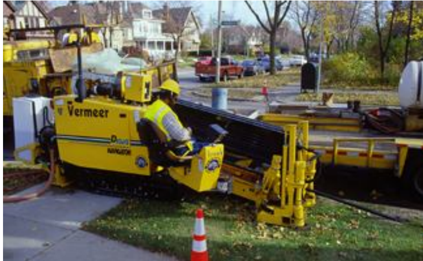
Figure #4: Horizontal Directional Drilling equipment
