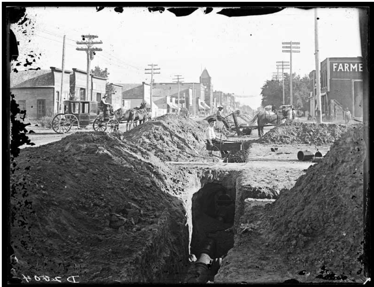
Figure #3: Sewer Construction Circa 1889
