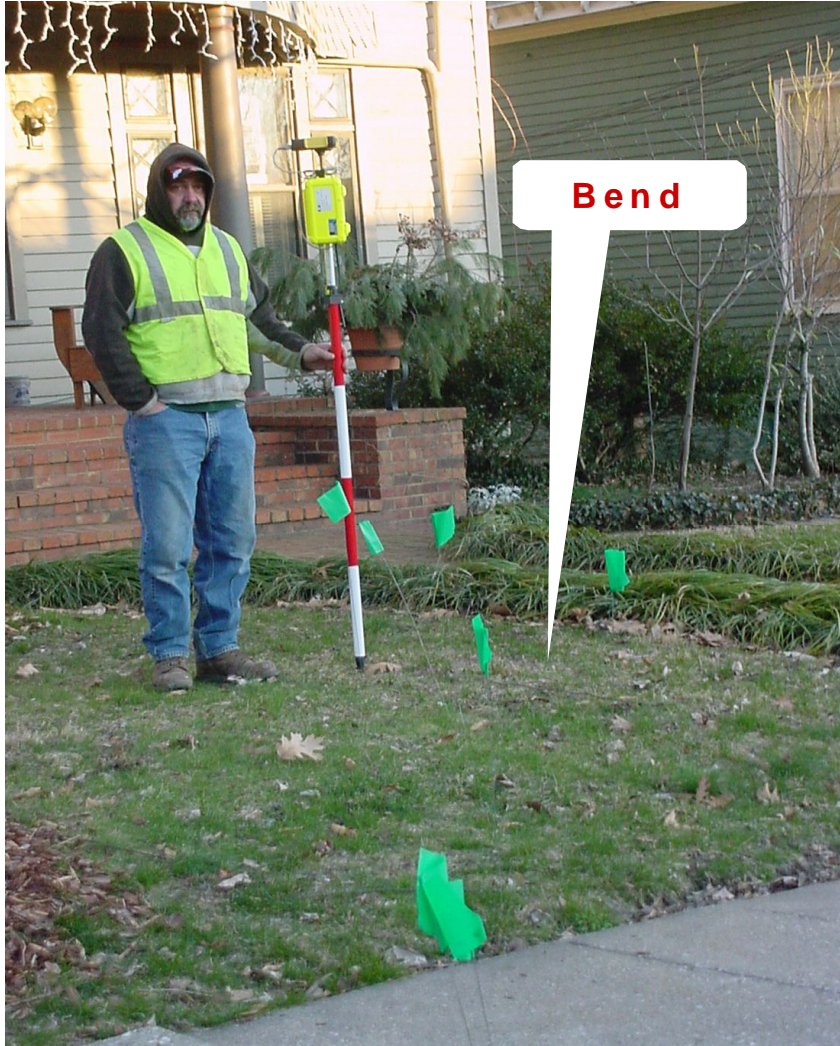
Figure 14 : CCTV Field inspector captures lateral line trace that has an unusual bend in the line
