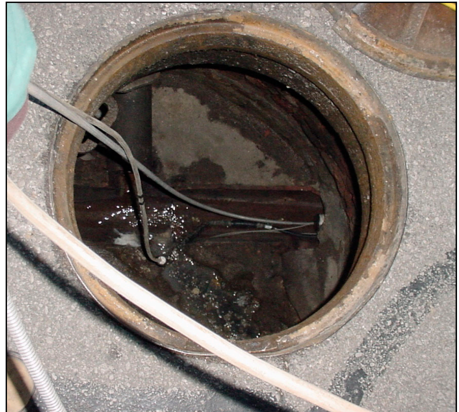
Traveling in Sewer Line
